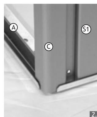
**(GB)** The screwed bottom section lies on a flat ground. As illustrated, put a side wall (S1)= panel with ventilation) into the short, left bottom element so that the ventilation is in the correct position. Fix the corner panel (C) at the left front corner (=side of the door threshold). Then, connect the middle of the corner panel with the side wall (S1) using two bolts, washers and nuts (nuts are always inside). Fix the back corner panel at the side panel the same way.
