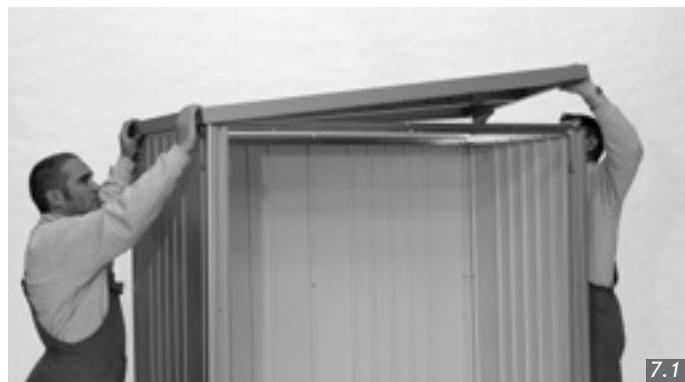
**GB** Now put the roof panel onto the side walls/ head sections and pay attention to the correct position of the roof panel as well as to the roof rest **F**. Screw the roof panel once at each corner and twice at the back side with the head section **B**.
